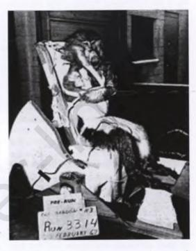
Fig. 10.7 The experimental research on the savannah baboon delivered the first knowledge of maternal and fetal physiology during and after motor vehicle accidents with belt restraint. Reproduced with permission from [90]
